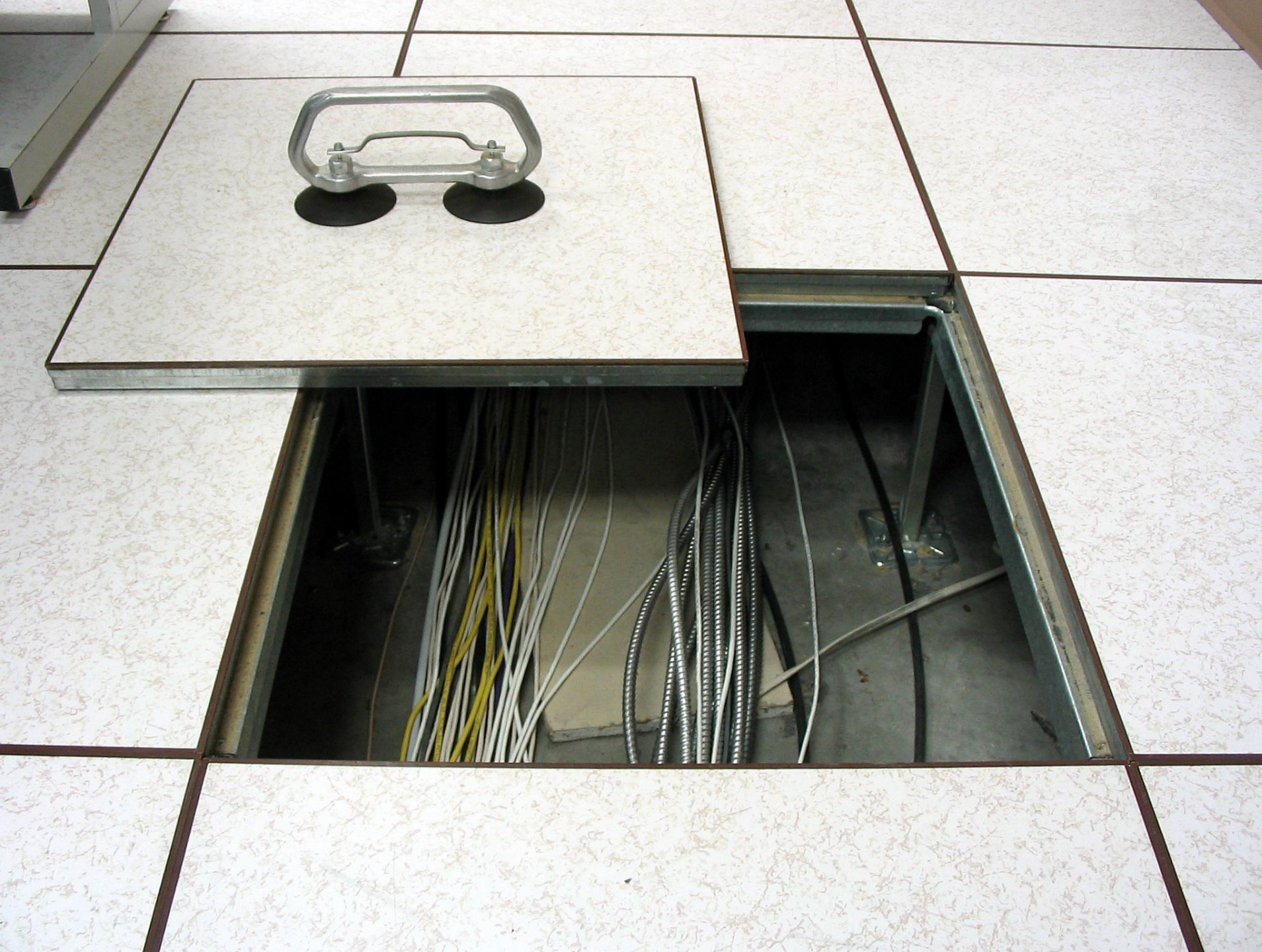
Raised floors to distribute cabling and cool air
