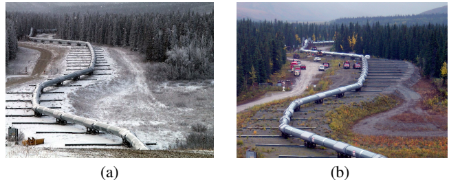
Fig. 1: Trans-Alaska Pipeline on slider supports where it crosses the Denali Fault [6]. This pipe suffered some damage, but no oil spills occurred. A large arc in the pipe can be seen in image (b), due to shortening of the zigzag-shaped pipeline trace in the fault zone.
